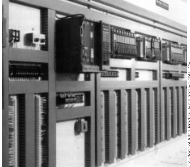
Figure 20-3. Placement of PLC components.
